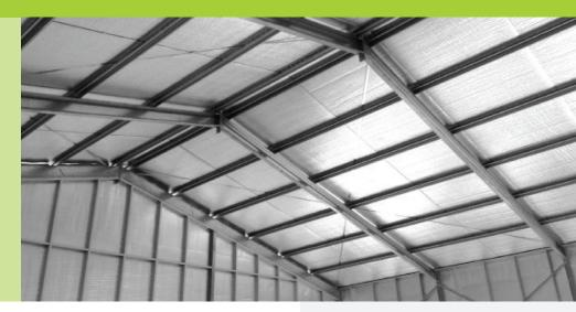
Trade Select™ ThermalLiner™ is an Extra Heavy Duty three-in-one reflective insulation, thermal break and Class 2 Vapour Barrier. Trade Select™ ThermalLiner™ is suitable for use in roof, wall and floor applications. Designed to manage heat gain and heat loss, Trade Select™ ThermalLiner™ offers superior thermal performance to conventional insulation, and reduces thermal bridging and conductivity between building elements.
