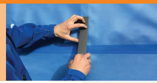
Ametalin ThermalBreak<sup>™</sup> Strips is an innovative dual-layer, high-density closed-cell XPE foam core self-adhesive strip. They are specifically designed to create an impressive R0.25 thermal barrier between steel framing and various cladding materials and roofing sheets.
