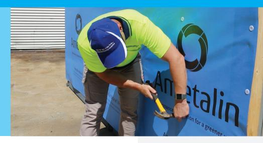
Ametalin Cap Nails<sup>™</sup> are a collated strip of 10 nails, each with an impact resistant polymer cap head. Designed to speed up installation time while providing over and above 20 x the holding power of plain nails or staples.
